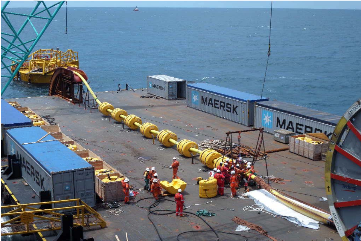
Subsea flexible flowline riser with buoyancy modules being run
